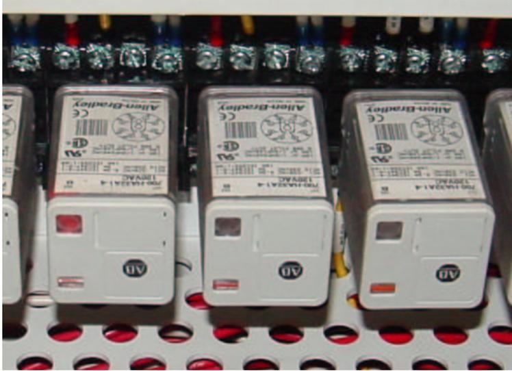
The relay units shown here are called "octal-base," because they plug into matching sockets, the electrical connections secured via eight metal pins on the relay bottom. The screw terminal connections you see in the photograph where wires connect to the relays are actually part of the socket assembly, into which each relay is plugged. This type of construction facilitates easy removal and replacement of the relay(s) in the event of failure.
