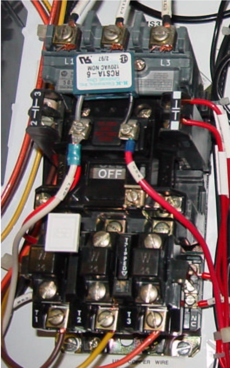
Three-phase, 480 volt AC power comes in to the three normally-open contacts at the top of the contactor via screw terminals labeled "L1," "L2," and "L3" (The "L2" terminal is hidden behind a square-shaped "snubber" circuit connected across the contactor's coil terminals). Power to the motor exits the overload heater assembly at the bottom of this device via screw terminals labeled "T1," "T2," and "T3."
